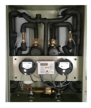
The Adveco HR001 Heat Recovery Box provides a convenient, packaged solution to recover refrigerant system waste heat.
