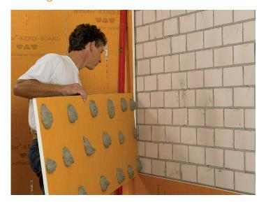
To be suitable for the installation of tiles in the thin-bed method with tile adhesive the substrate must be completely level and made of an appropriate, moisture resistant material. However, walls are frequently covered with a gypsum plaster coating as part of the construction. Plaster is not an ideal substrate for tile coverings, especially in high moisture areas.
