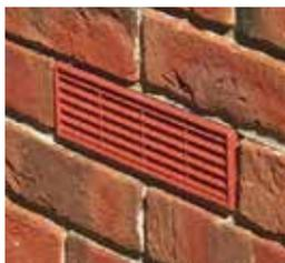
Radon evacuation from structure via Cavibrick located under Radon cavity barrier level.
