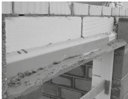
Uniformity and consistency can be difficult to achieve using soft roll DPC but with a preformed Type C Cavity tray the angle and dimensions can be specified and maintained.
