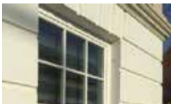
Type SDC water evacuation is in place with the discreet outlets set back in the rendered reveal.
