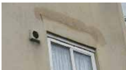
Weeps omitted so water is trapped on DPC between stopends
