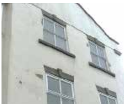
Water has penetrated causing render to fail throughout elevation.
