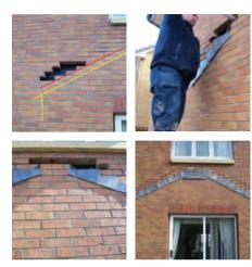
In remedial applications where an existing DPC has failed or been omitted, installation follows the identical procedure.
