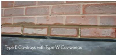
Type E Cavitytrays with Type W Caviweeps
