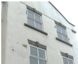
Water has penetrated causing render to fail throughout elevation.
