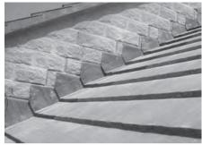
Multi-course Cavitrays installed in 150mm (6inch) steps. In this example trays have been inserted into an existing wall, demonstrating masonry removal is minimal.
