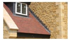
Multicourse Regular Wide Front to Back Dimensions. The natural hamstone is built against a concrete backing black resulting in an external leaf of 250mm thickness beyond which is the cavity. Thus the trays have extended front to back dimensions.
