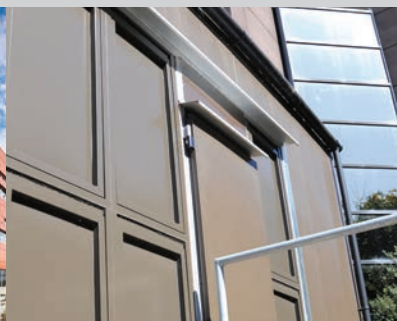
C/S Explovent® Explosion Venting Systems
