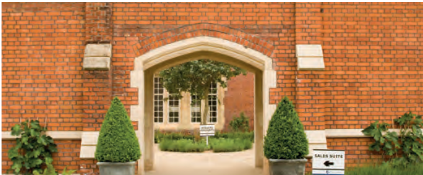
Replacement arch on restoration project
