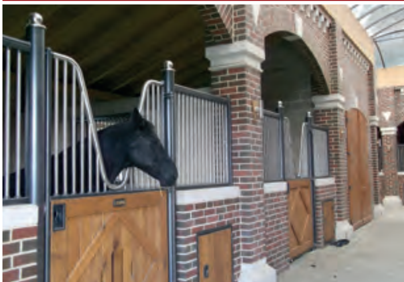
Extensive use of cast stone on stunning equine facility
