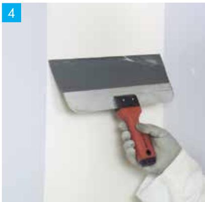
Applying the second coat of Knauf Joint Cement Premium.
