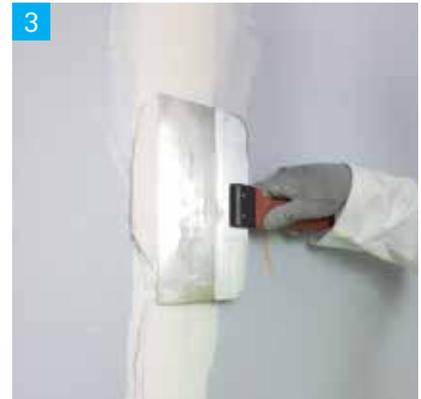
Applying first coat of Knauf Joint Cement Premium.
