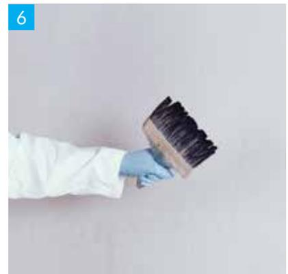
Applying Knauf Wallboard Primer for Tape & Jointing system only.
