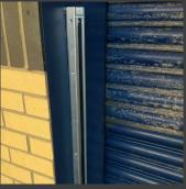
rails are available in two forms. either "reveal fix" which means fixing in between the reveals/ brickwork of the doorway or "face fix" which means fixing onto the face of the brickwork.
