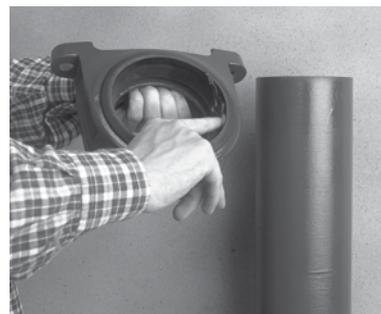
2. Push coupling over the end of pipe/fitting, ensuring the central register is abutted against the spigot edge evenly. If the coupling is eared, fix to wall using anti-corrosion coach screws or similar.
