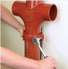
Check alignment of assembly before tightening the bolts. Coupling bolts on all sizes are M8 and require special Allen socket adaptor (6mm) EF102, together with a ratchet spanner EF100. Alternatively use a time saving power tool.
