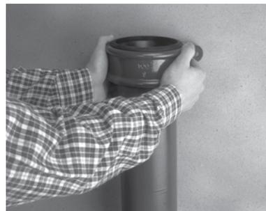
3. Push the second pipe or fitting into the gasket again ensuring that the spigot is abutted against the central register. Timesaver Heritage couplings eared/plain can be fitted to most fittings within the 50, 75 and 100 diameter ranges (see table page 192).
