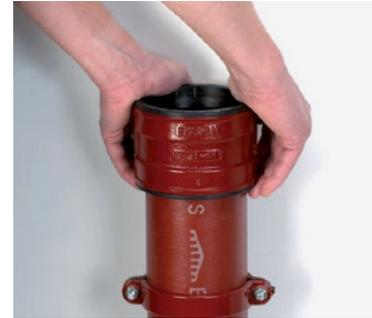
2. Push joint over the end of pipe, ensuring the central register is abutted against the spigot edge evenly.
