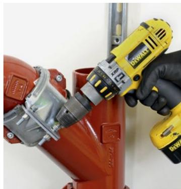
2. Insert the four screws to fix the two parts together loosely.
