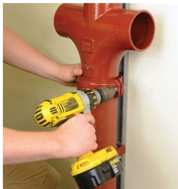
**Note:** Bolts should be tightened until a suitable resistance is achieved if using a torque wrench if using a power drill or ratchet spanner 20Nm.
