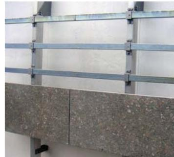
Stone installation made on to stainless steel channel system. T31 undercut bolt is used with specially designed anchors. T31 bolt is fastened on to the anchor using contra nuts.
