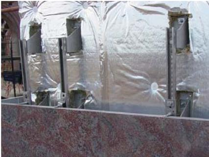
Sub channel support system designed to bear heavy loads at projection sizes exceeding 40 cm. Stone panels are installed using T31 undercut bolts.
