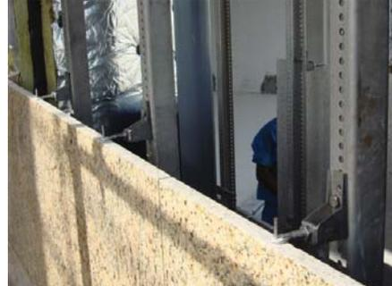
Stone installation made on to stainless steel channel system. T31 undercut bolt is used with specially designed anchors. T31 bolt is fastened on to the anchor using contra nuts.
