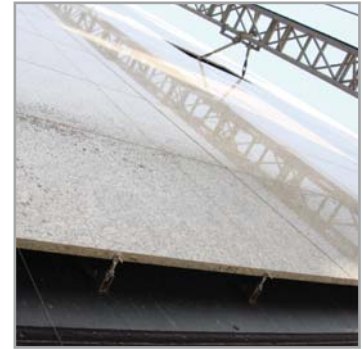
• AXO body anchors are used to install stone panels at horizontal joints to concrete substrate
