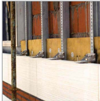
• HA L anchors are used to install stone panels to backing wall at horizontal joints. On the left picture, anchors are attached to steel channel. On the right picture, anchors are attached to concrete substrate.
