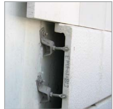
• Z anchors are used to install stone panels to concrete substrate. On the left picture horizontal joint application. On the right picture vertical joint application.
