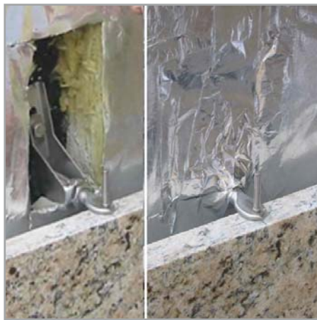
• Z anchors are used to install stone panels to concrete substrate. On the left picture horizontal joint application. On the right picture vertical joint application.
