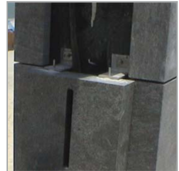
• HA L anchors are used to install stone panels to backing wall at horizontal joints. On the left picture, anchors are attached to steel channel. On the right picture, anchors are attached to concrete substrate.
