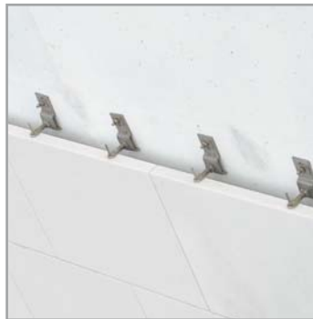
• Z anchors are used to install stone panels to concrete substrate. On the left picture horizontal joint application. On the right picture vertical joint application.
