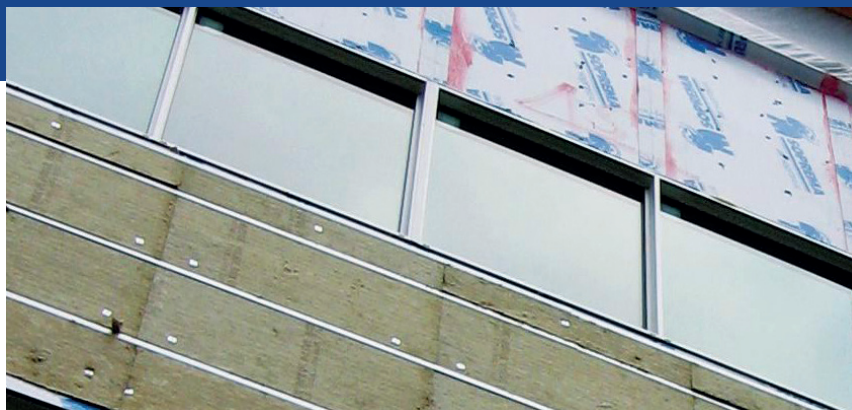
Exterior insulation installed in-between steel z girt cladding support attachment resulting in exterior insulation that is not continuous and does not meet energy codes (Source: Roxul, Inc.)
