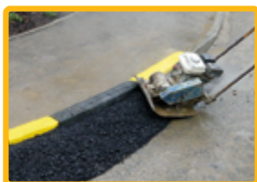
Haunch with temporary tarmac
