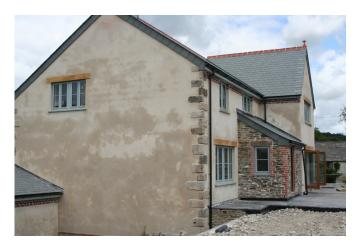
The second coat is the straightening coat, so after application the work needs to be ruled/staffed off, to further straighten the work to produce the desired level of finish (if necessary).
