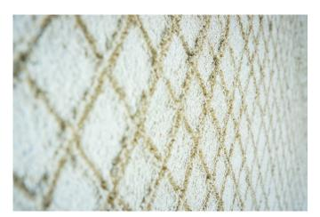
Remember: The scoring should not be such as to tear the render off the wall.
