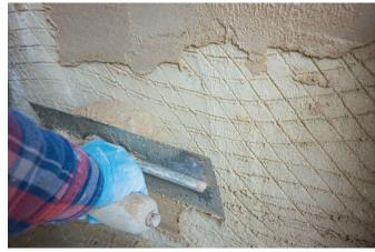
Alternatively, apply the first coat as normal using a laying-on trowel, using even pressure to 'press' it on or into the wall. Lime mortars are extremely cohesive but require more effort than for cement bound render, requiring greater pressure to press the render onto the surface (aided by the pre-damping).
