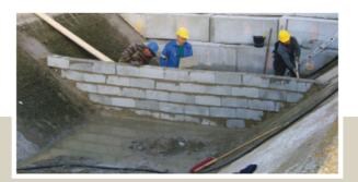
Natural coment allows the rapid return to use of hydraulio structures
