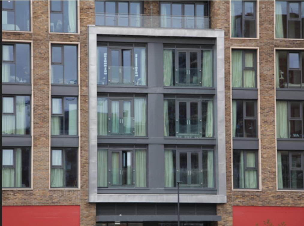
Fire performance, chemical composition and resistance to pull-out loads were all factors considered by one of the leading national contractors in the selection of Magply MgO boards for the cladding build-up on four apartment blocks in Bristol.
