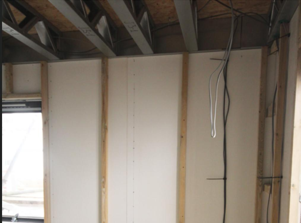
The task of adding an extra floor to an apartment building in the heart of Brighton has seen the 12mm version of IPP Ltd.'s Magply boards employed in a variety of applications, both internally and externally: highlighting the well proven MOS product's fire performance, weather resistance and overall economic benefits.
