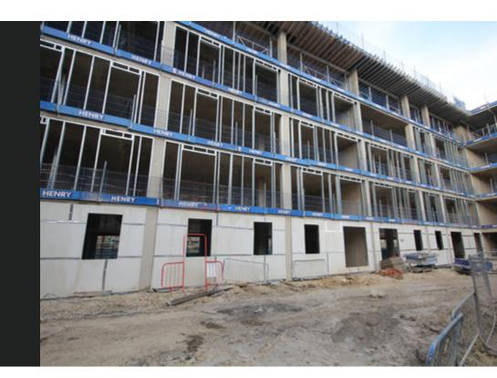
Hundreds of square metres of 9mm Magply boards are currently being installed on an apartment development close to Reading's commercial centre, after the specialist package contractor involved proposed the high performance MgO panel as an alternative to the original product specified, representing a value engineering solution.
