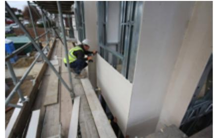
While in respect to this project, the UniFrame system includes diagonal ties which are tensioned on site, Magply is often used by timber frame manufacturers to take the racking loads for their buildings as well as to provide fire protection in close proximity to other properties.
