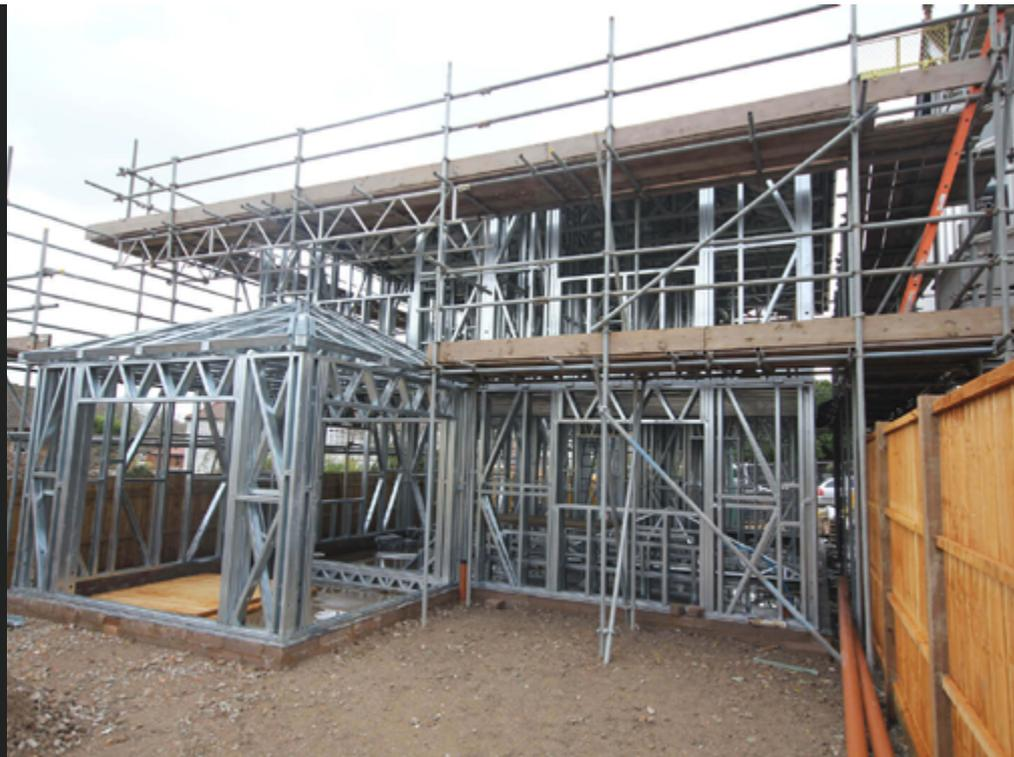
A cutting edge residential project in Essex is making use of Magply boards for both the internal lining and exterior cladding treatment to an innovative lightweight steel framing system, demonstrating the widely specified fire resistant product's multiple attributes.
