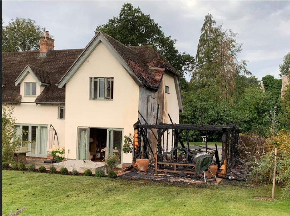
A potentially catastrophic blaze, which consumed the garage containing a parked vehicle adjoining a £1M house in rural Surrey, was stopped in its tracks thanks to the use of 12mm A1 non combustible Magply being chosen as the render substrate board on the contract, the property was constructed using a Structurally Insulated Panel system construction (SIP) with A1 non-combustible Magply being used on the exterior of the building as the substrate panel for the proprietary render system.
