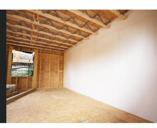
A 'shell & core' style apartment development in one of South London's up and coming districts is making use of Magply boards' fire resistance and other performance characteristics, as the lining to a bespoke timber frame package.
