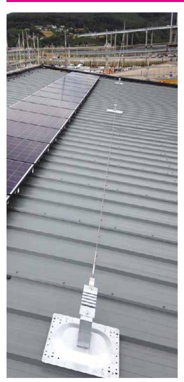
The **KEELINE** horizontal lifeline system is designed to provide safe access to any area of a roof by allowing workers to be permanently attached to the line at all times and be able to freely move around the roof surface. The system utilises 8mm grade 316 stainless steel wire and allow spans of up to 12m between posts and can be utilised by up to three users at any one time.
