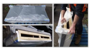
Lift the canopy upright and cut open the packaging at the rear. Taking care not to damage the finished surface slide the packaging off the canopy. Only fully remove the canopy from the packaging when fitting is imminent.
