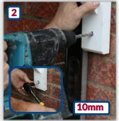
Mark and pre-drill 4 holes with a 6mm (x2) and 10mm (x2) bit. Position the bracket level with the door head, or where desired, ensuring the width between both brackets won't exceed 1200mm. Using the pre-drilled holes, drill through the bracket and into the wall (10mm bit), ensuring it is level vertically. Secure using 2 SXR 10x80 fixings (see inset).
