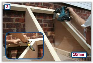
Using the pre-drilled holes, drill through the frame into the wall, using a 10mm bit (x4). Fix with 4 SXR 10x80 fixings.
