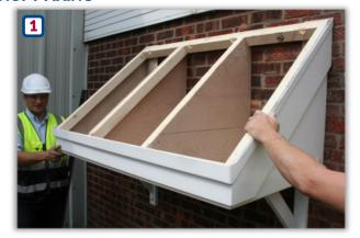
If required, apply mastic sealant to the rear of the canopy. Then carefully lift and place onto the gallows brackets.
