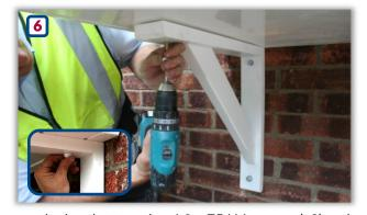
Secure the bracket to using  $6.0 \times 75/46$  screws (x2) and suitable white cap (see inset). Repeat for other bracket.
