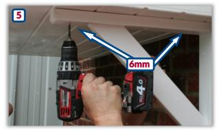
Using the pre-drilled holes, drill through the bracket and into canopy underside. Repeat for other bracket.
