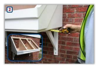
Centre the canopy, ensure an equal distance from each bracket to the canopy edge and push to the wall.
