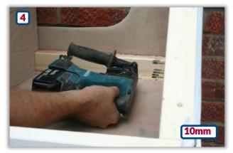
Using the pre-drilled holes, repeat as step 3 with the 4 fixing points on the lower part of the frame.
