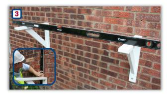
Ensure the second bracket is level horizontally and equidistant from the door frame as the first (not exceeding 1200mm). Using the pre-drilled holes, drill through into the wall (10mm bit) and secure bracket as before (2 SXR 10x80 fixings), ensuring it is level vertically (see inset). The brackets are now ready to receive the canopy. Copyright © 2016 Brickfab Ltd
