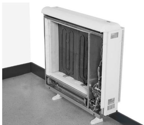
10.- Place the heating elements back into their original position. Place the other two rows of storage bricks with the flat side facing out and always on the heating elements supporting tabs.
