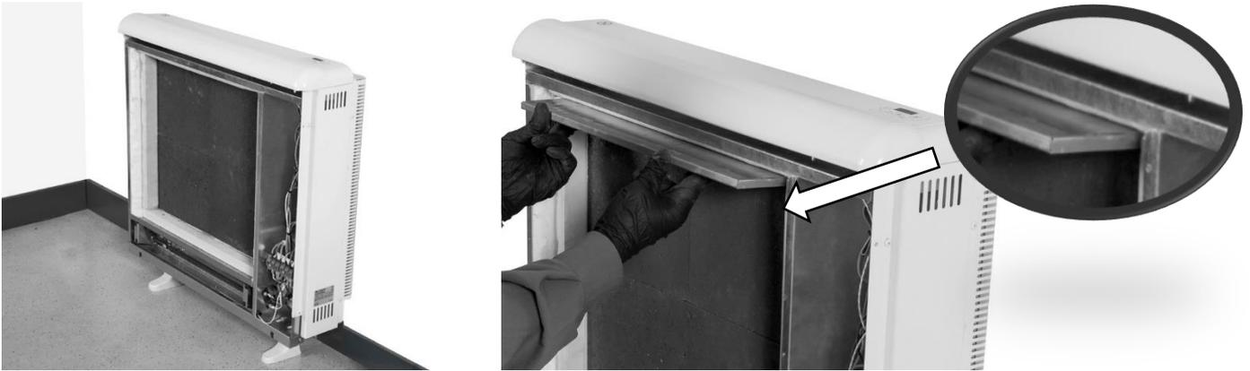
12.- Place the third row of storage bricks with the flat side facing out.
