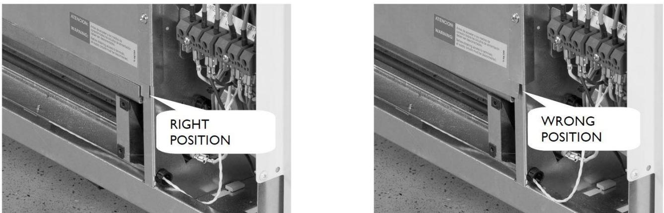
14. Replace the front panel. When refitting the exterior front panel, align the 2 metal upper pegs on the heater with holes in the exterior panel. Push the top up into place and push the bottom in, then refit the screws.
