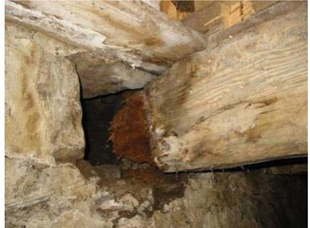
*Fig. 1* Decayed floor joint in wall pocket
