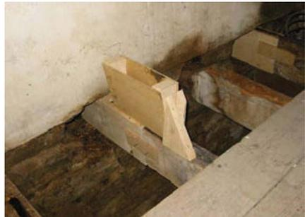
*Fig. 6 Header box to assist pouring of TG6*
