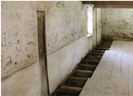
*Fig. 2* Sufficient floor boards removed for access
