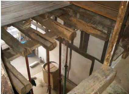
*Fig. 2 Propped floor joists with decay removed*
