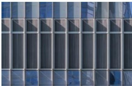
Horizontal blade louvres are the most common, with both continuous line and visible mullion options available.
