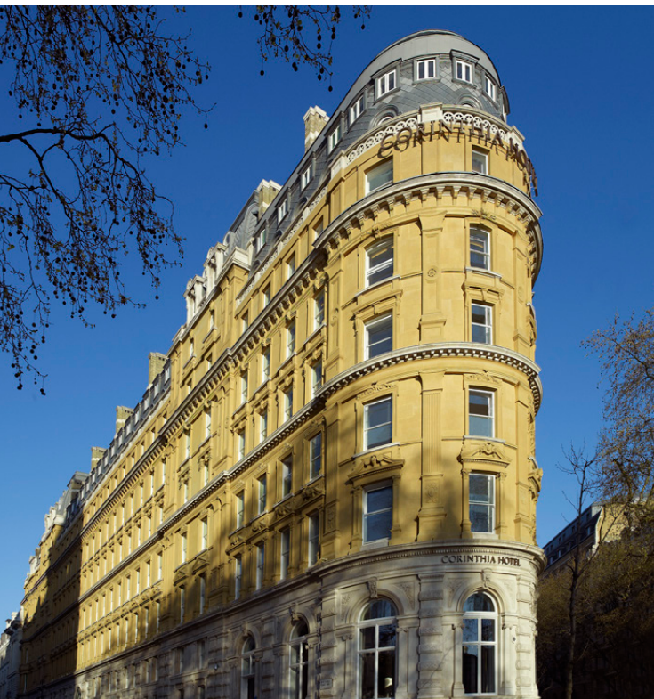
Aquasystem Installation Corinthia Hotel London
