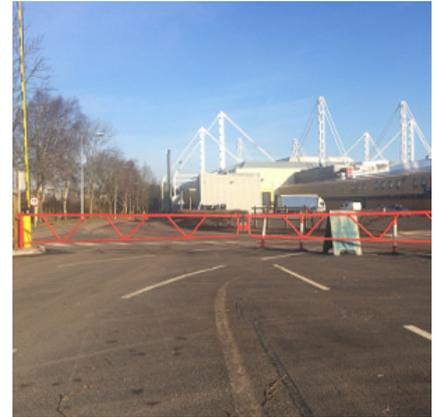
The AUTOPA Double Swing Gate is a manually operated, ideal for securing entrances to large industrial and commercial sites. Gates can be locked in both the open and closed positions. Additional catch posts and padlocks are available separately if required.
