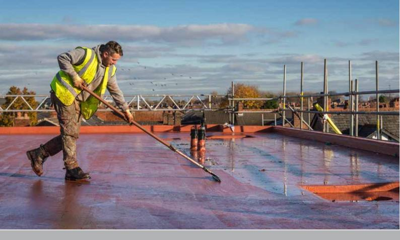
Liquid roofing is a technology unlike any other. It offers significant advantages over all types of conventional and sheet roofing materials.
