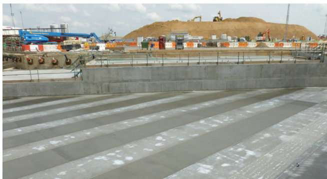
Intercrete 4841 is simple to apply and is an effective barrier to chloride ions
