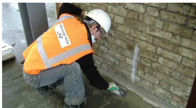
Intercrete 4823 is fibre-reinforced for added strength and durability
