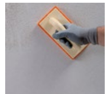
Finishing off the surface with a sponge float
