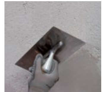
Application of fine texture skimming mortar
