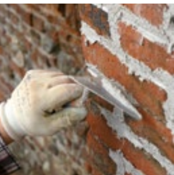
Pointing between brickwork
