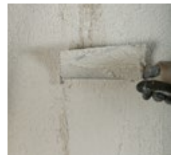
Application of dehumidifying render
