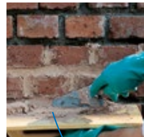
Pointing between brickwork
