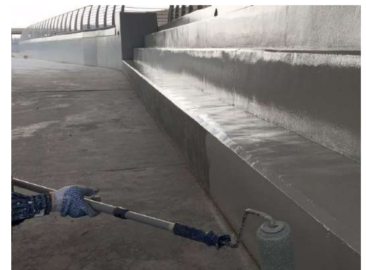
Apply the protective coating system
