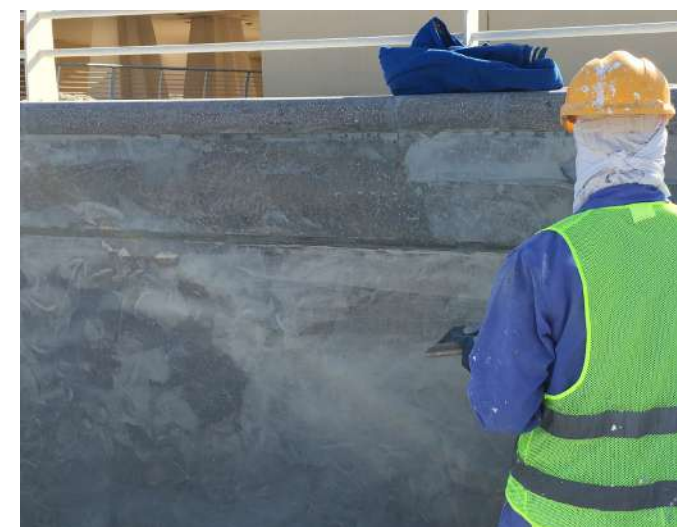
Small scale face filling between coats
