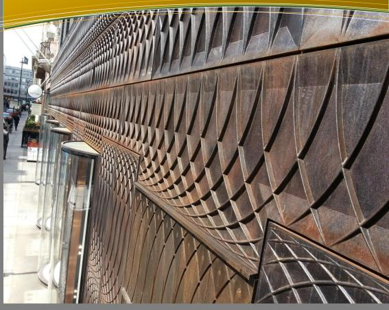
FSE worked together with a number of architects from 6A and were able to produce a number of large cladding pieces in SG Iron to front the latest Paul Smith shop.
