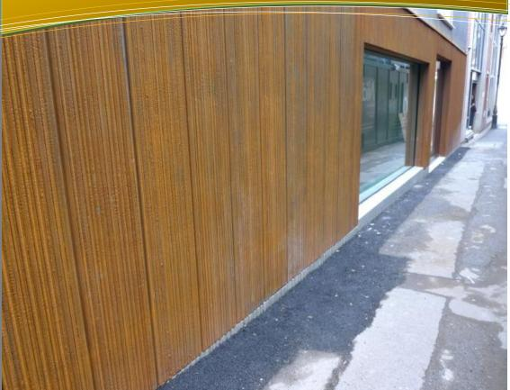
FSE worked together with an architect, showing the capabilities of casting and pattern modifications available and were able to cast a very unique form of cladding in Cast Iron.
