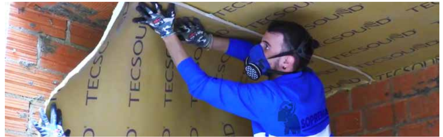
APPLICATION OF TECSOUND® FT IN FALSE CEILINGS
