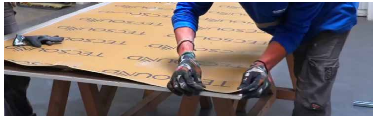
APPLICATION OF TECSOUND® SY IN DRYWALL PARTITIONS
