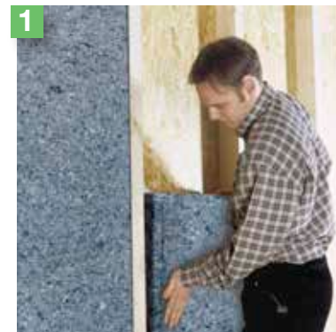
Laying the insulation in walls, timber frame
