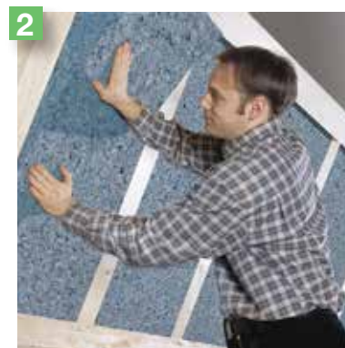
Laying the insulation in attics
