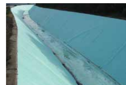
Irrigation channel. Alagón.
