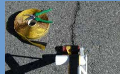
Asphalt crack filling (Stratos R2 with installation tool)
