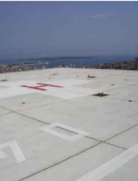
Kerosene resistant joint on a heliport (Stratos R4)
