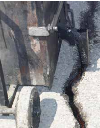
Hot asphalt crack filling (Transifal C40)
