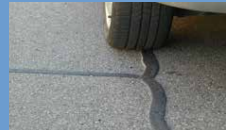
Cold asphalt crack filling (Stratos R2)
