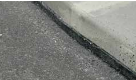
Concrete/asphalt junction (Stratos R1)
