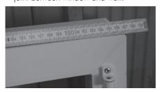
4. Select the dimensions of the tape according to the fitting depth of the window frame and the recommended range of the joint size. (see carton label).
