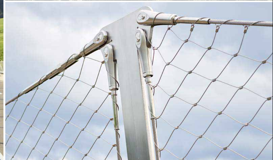
Hundwilertobelbrücke, Appenzell AR (CH)
