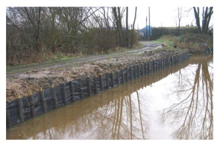
**Nicospan** is a product for vertical bank protection. It can provide a high-quality and very economical form of erosion control. Nicospan is a prefabricated, double weave revetment fabric made from strong UV stabilised monofilament yarns that are heat sealed to form a series of open pockets each having a width of 220mm so that 75mmØ/100mmØ posts can be placed into them.
