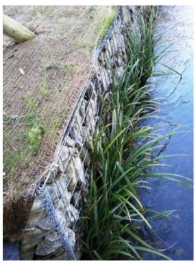
Verdant Solution's unique system incorporates pre-established vegetation within the face of stone filled gabions. Well rooted vegetation pre-grown in coir modules is an integral part of Verdant Solution's Green Systems of erosion control. We help Clients to incorporate well established vegetation at the waters edge even where the projects require hard engineering solutions.
