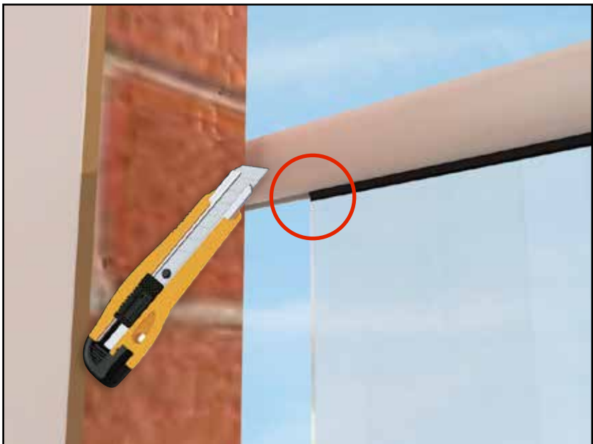
15. Trim off excess rubber.
