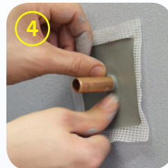
4. Apply Pipe Sleeves
