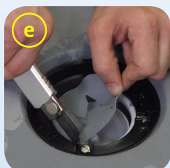
e. Cut away the excess sleeve inside the ring
