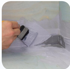
3. Apply Pre-formed Corners (internal or external)
