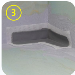
3. Apply Pre-formed Corners (internal or external)
