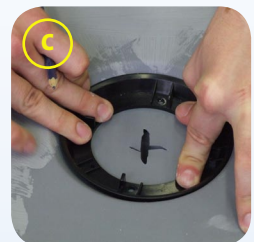
c. Push down on clamping ring and mark screw holes
