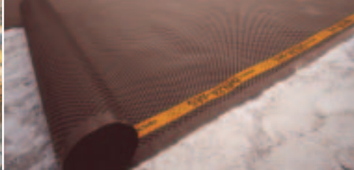
Overlaps should be 20 cm minimum.
