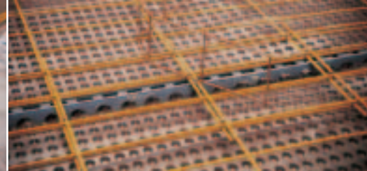
Reinforcement-mesh spacers are safely held in place.
