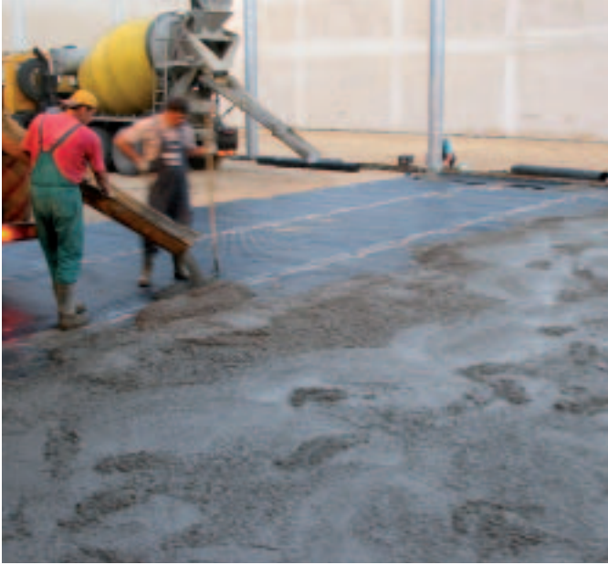
DELTA®-MS Sub-base Course offers a high degree of safety when applied under fibre concrete.
