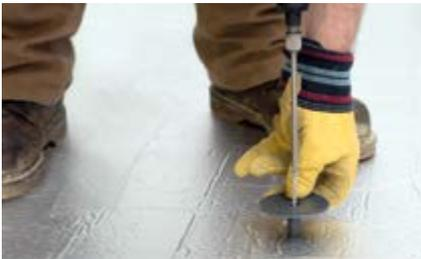
Where installers prefer to mechanically fixed insulation to the deck but adhere the waterproofing membrane, EJOT has developed a unique 75mm diameter tube-washer to meet SPRA guidelines for part-mechanical / part-adhered hybrid installations.
