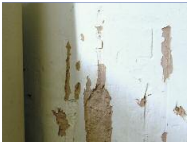
Lightly damaged areas deteriorate quickly, making proper cleaning difficult
