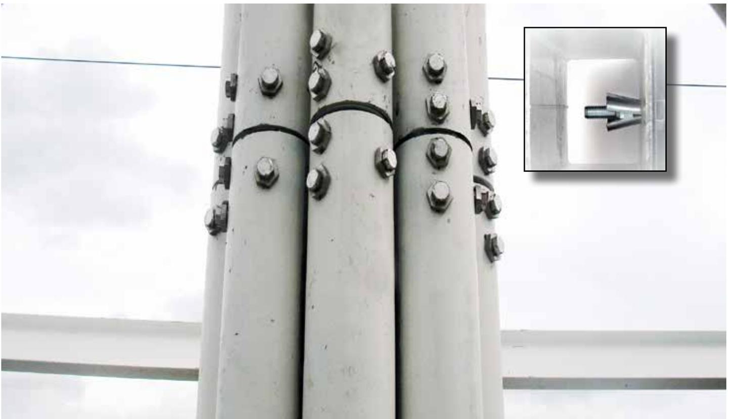
Stainless Steel **BOXBOLT** fixings were used to create a splice detail (tube within tube) to create the neat looking steel structure that was then glazed to create a sheltered area for transit passengers. The **BOXBOLT** detail allowed for the neat tubular joint to be made without the need for expensive labour or equipment on site.
