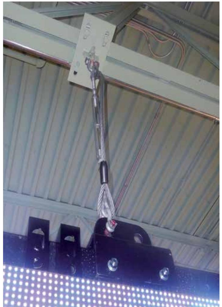
Our BK Rigging clamps were used to provide a suspension point to the roof trusses in a shopping mall. The suspension points were used to hang heavy duty wire that suspended a large LED display screen for the shopping mall customers. The use of our BK rigging clamp assembly avoided the need to break the painted surface of the existing steel and also allowed for final adjustment on site.
