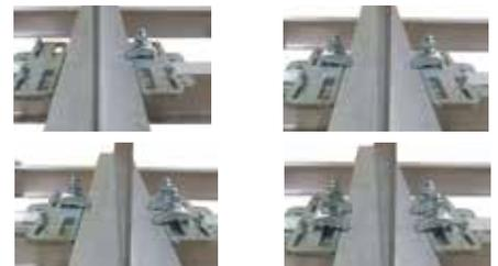
**STEP 4** - The front and back edge of the clamps should run parallel with the steel sections.
