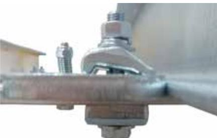
**STEP 5** - Hold the head of the bolt with a standard wrench and tighten the nut with a torque wrench to the recommended torque stated above. Repeat this for all four bolts.
