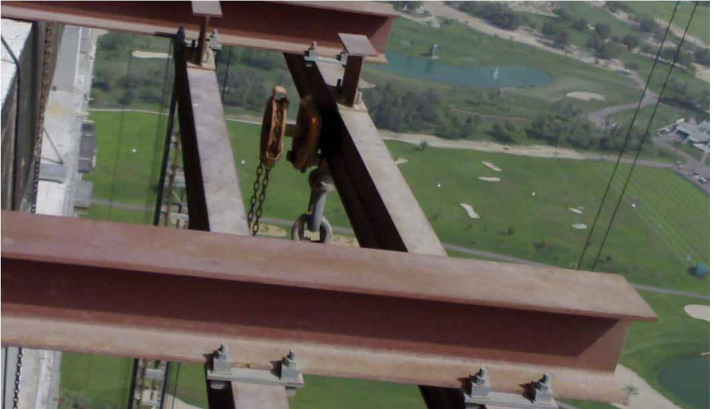
**BEAMCLAMP** is an extensive range of clamping products designed for making steel to steel connections without the need for drilling or welding. The clamping system gives the specifier the peace of mind that once the connection is made it has a guaranteed safe working
