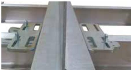
**STEP 3** - Insert one set of clamps through each corner ensuring they are positioned as in step 4.
