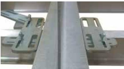
**STEP 2** - Rotate the open side of the plate around the sections so that the frame is complete.
